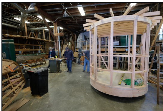
Top: volunteer Bill Isaacs works on the Hyak build (photo courtesy of Shaun O'Berry). Below: the finished wheelhouse will be roughly 8' x 7'-6".
