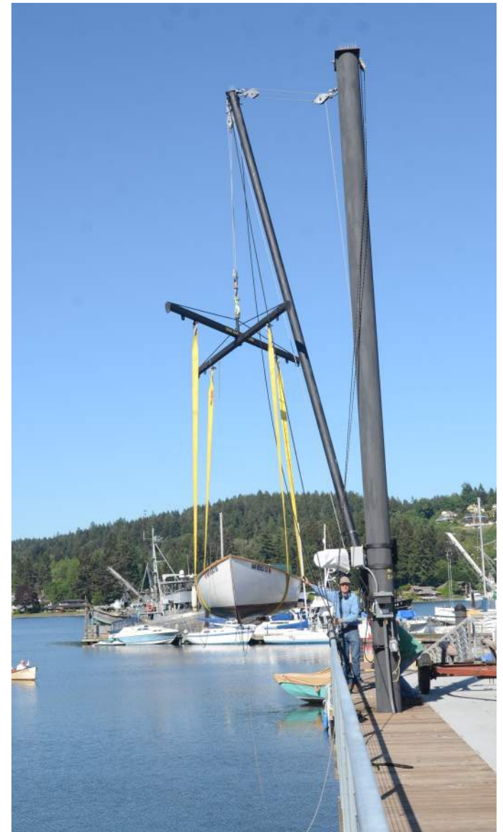
Completed in 2016, the mast and boom on the Eddon Boatyard dock enable the BoatShop to lift small vessels from the water.
